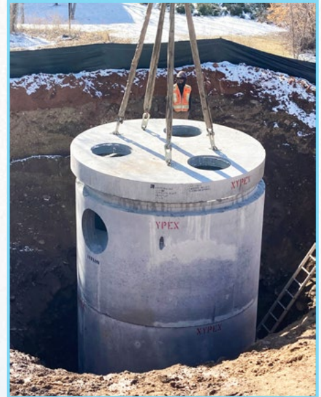
Step 3: Place top slab with access holes.
