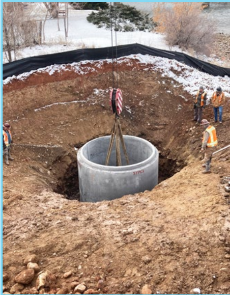
Step 1: Install the base section.
