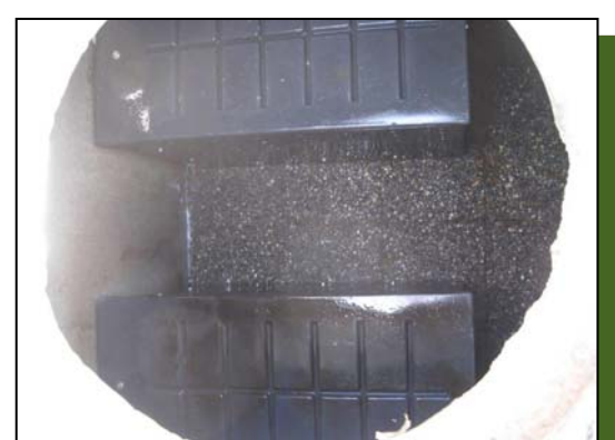
Fully cleaned separation chamber.
