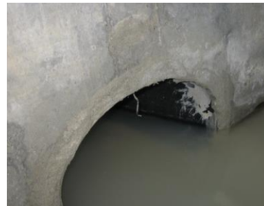
Example of a GOOD pipe installation. Pipe flush with the internal wall of the structure, clean grouting, and proper position.
