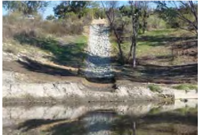
FIG. 5. Construction of the riprap waterfall into the wetland basin.
