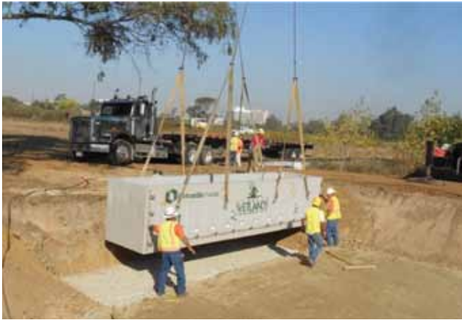
FIG. 4. Dropping of the precast box during construction of the WetlandMod system.
