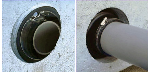
Example of appropriate pipe connection using a Kor-N-Seal. Note that the pipe does or connector does not protrude past the structures inside wall.
